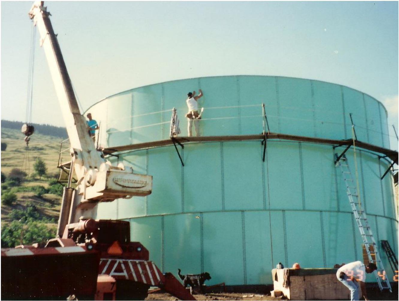
STATE OF HAWAII KULA HOSPITAL, INSTALLATION OF TWO 300,000 GALLONS ABOVE GROUND WATER STORAGE TANKS
